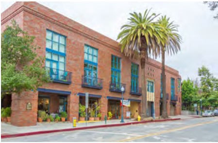
Mission Meridian Village. Courtyard housing, single-family houses, duplexes and mixed-use lofts.
